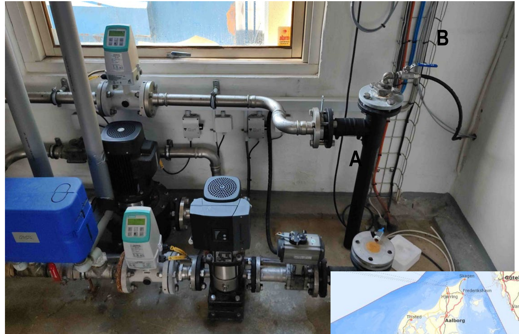
Fotos from the room next to where the GreenCat tank are at the Innovation Garage. The polluted water comes into the facility through pipe A and the water to the greencat-project are taped from B, before the remediation-facility marked with a C,
