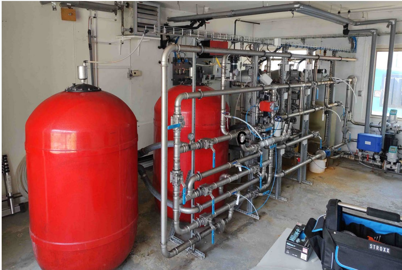
Fotos from the room next to where the GreenCat tank are at the Innovation Garage. The polluted water comes into the facility through pipe A and the water to the greencat-project are taped from B, before the remediation-facility marked with a C,
